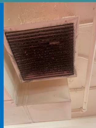
Damaged and dirty air filter
