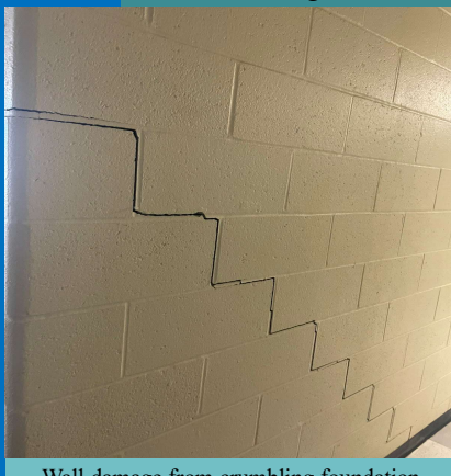
Wall damage from crumbling foundation
