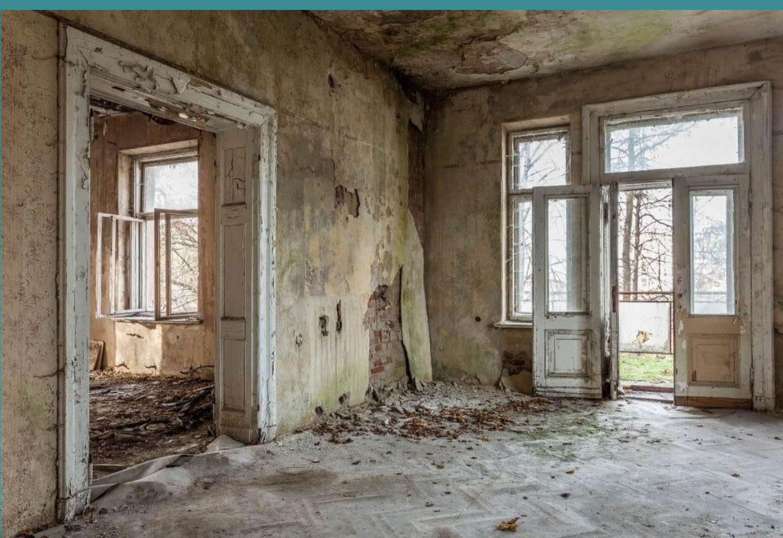
New Orleans Interior Demolition Services | Big Easy Demolition https://www.bigeasydemolition.com/service/new-orleans-interior-demolition/
