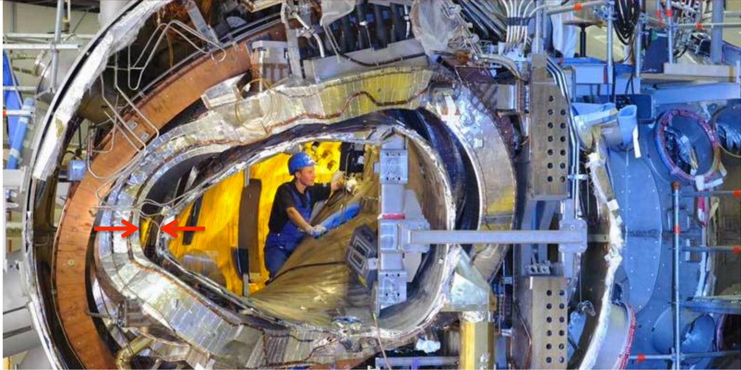
“Lesson 1: A lack of generous **margins, clearances and reasonable tolerance levels** implies an unnecessary increase of the complexity and leads to late design changes. This has a strong impact on schedule, budget, man-power and potentially sours the relationship to funding bodies.”
