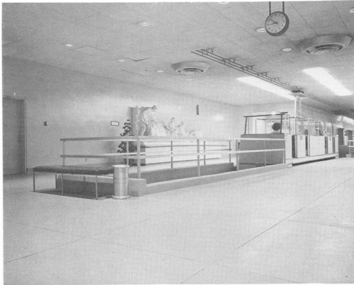
FIG. 1. U.S. Capitol—Rayburn House Subway Loading Platform.
