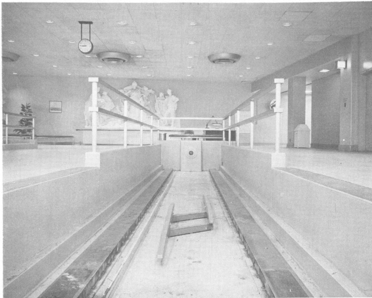
FIG. 2. U.S. Capitol—Rayburn House Subway Overshoot Area. The end of the overshoot is 6.1 m (20 ft) beyond the normal stopping position of the subway car.
