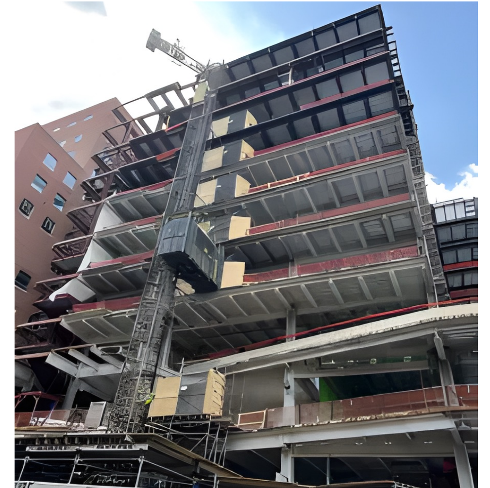
North tower being topped out
