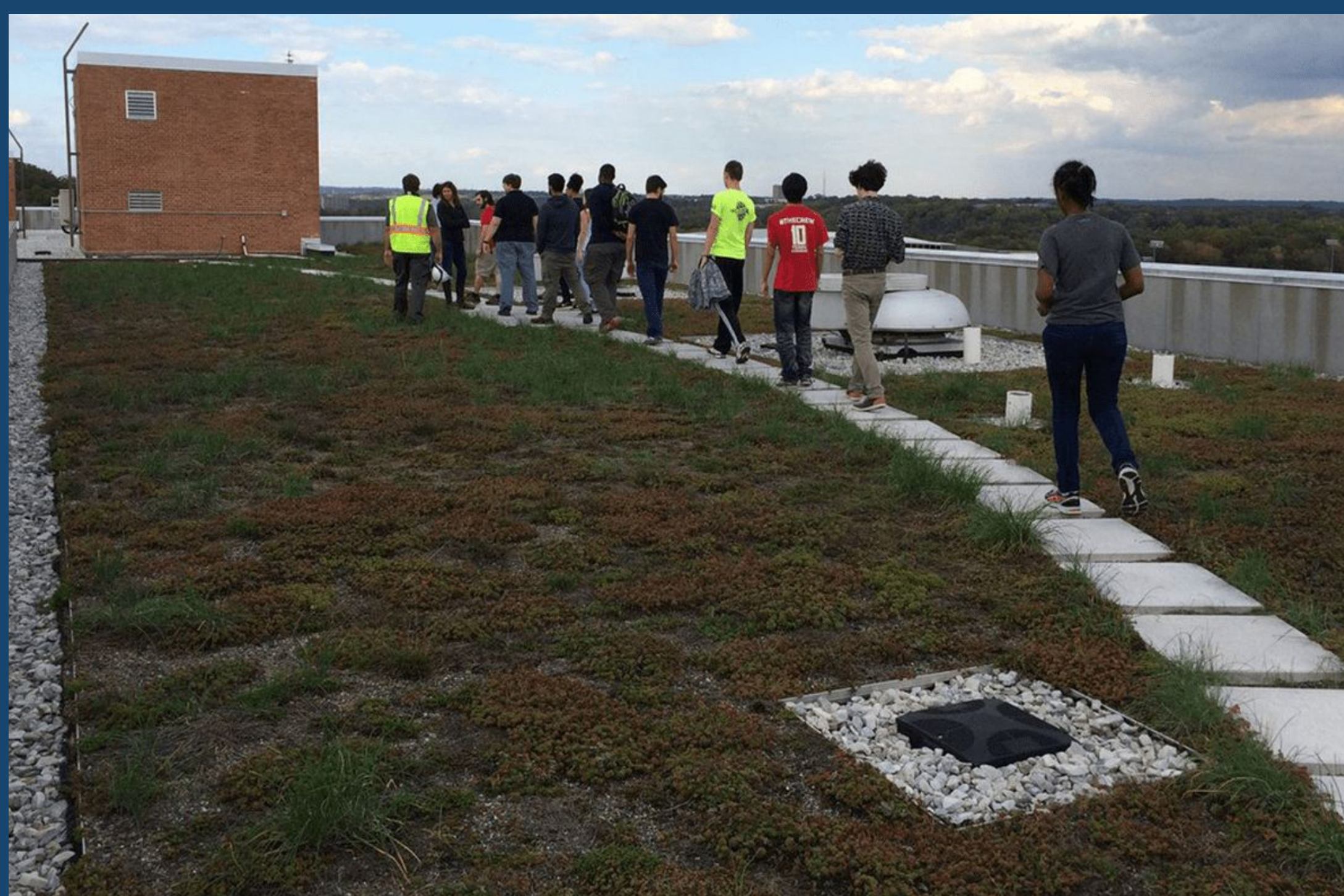
UMD's Stormwater Management and Maintenance Inspector, Michael Carmichael, gave us a tour of the water infrastructure around UMD, including Cumberland Hall's green roof displayed above. Image from SustainableUMD ( https://sustainability.umd.edu/topics/water/water-initiatives )
