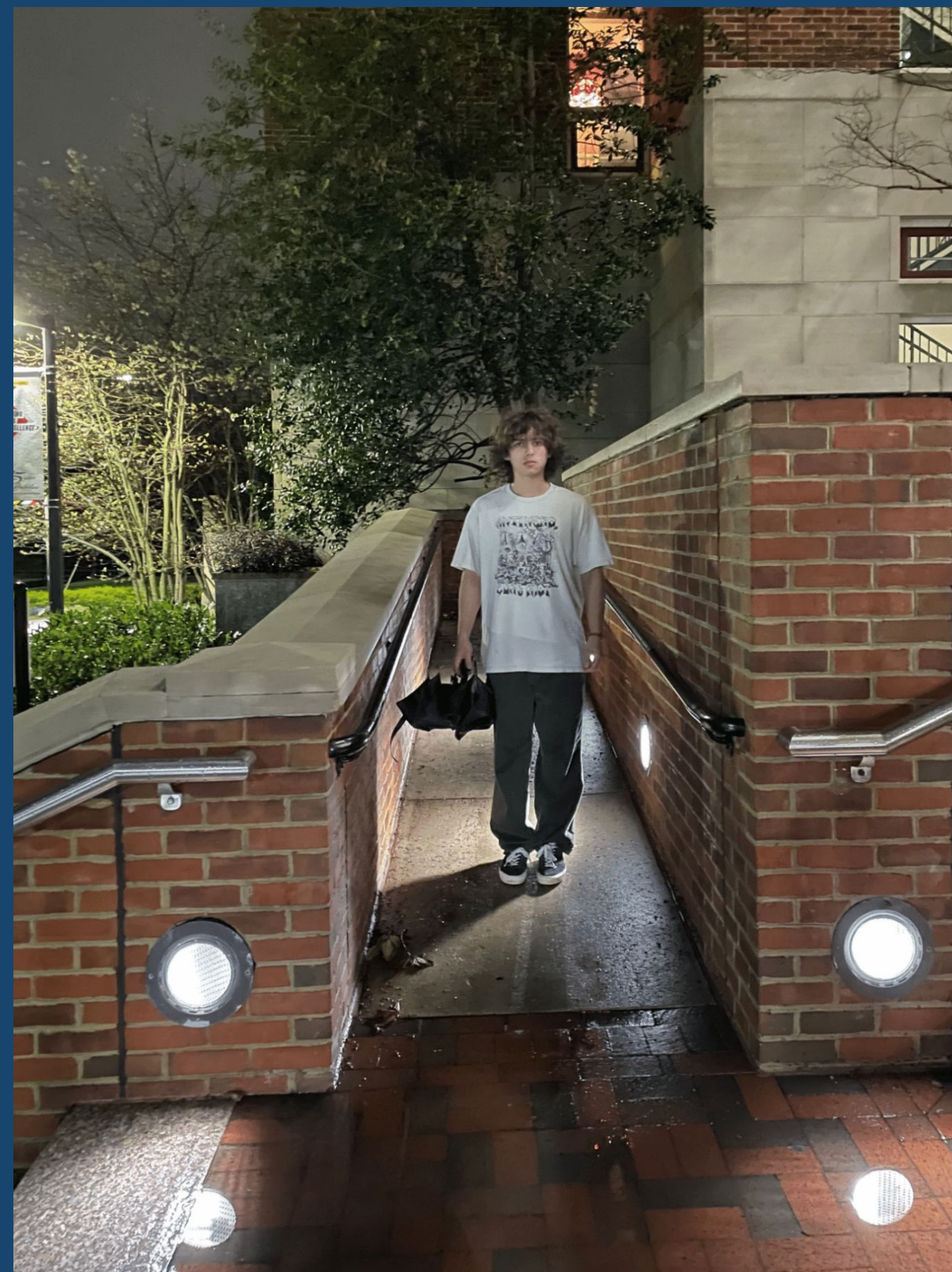
I am shown standing to show the width of a wheelchair accessibility ramp in front of Van Munching Hall. My aim was to highlight how the ramp was too narrow to comfortably accommodate a wheelchair user, and the photo was submitted for one of the journal assignments we had for the class.
