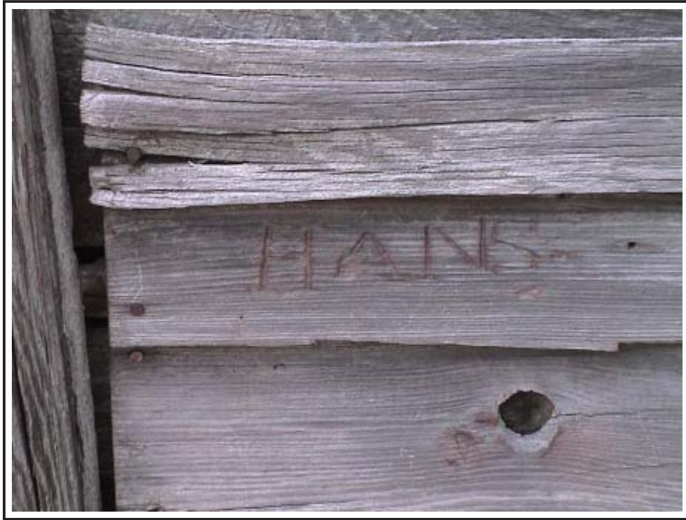
Figure 4.6. "Hans" inscribed into weatherboard on west side of front facade, Goulson frame house, ca. 1880.
