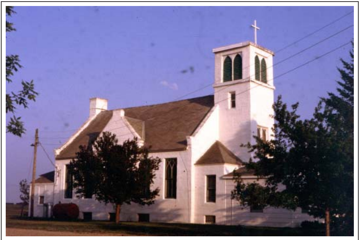
Figure 2.9. Mandt Lutheran Church, Mandt Township, Chippewa County, MN.
