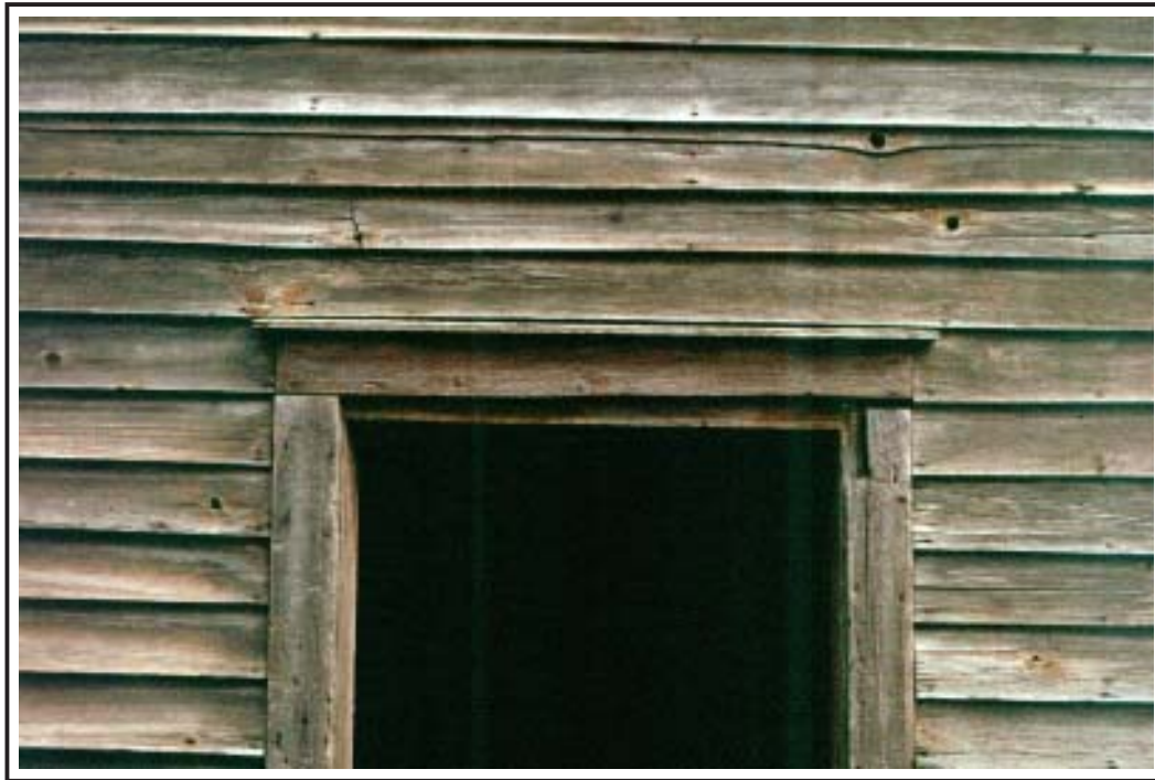
Figure 4.4. Detail of the front door trim, Goulson frame house, ca. 1880.
