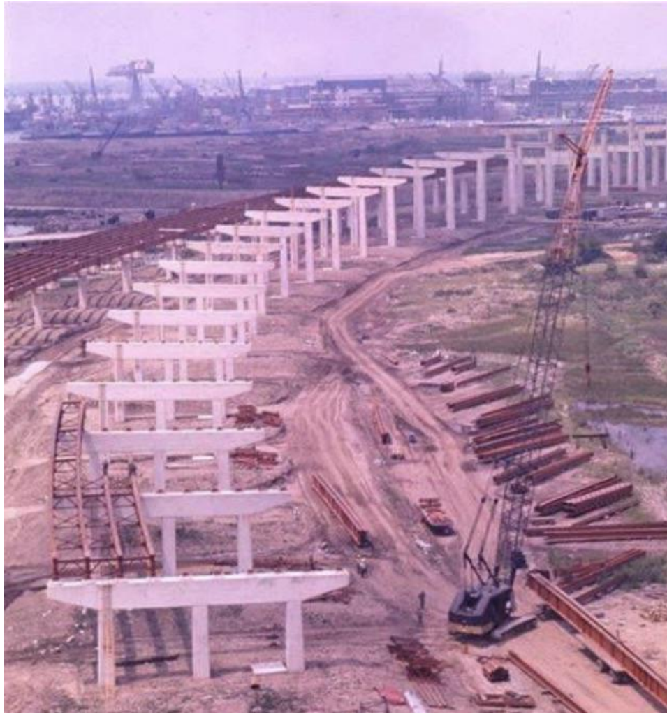
Construction of I-95, near Philadelphia, circa 1970.
